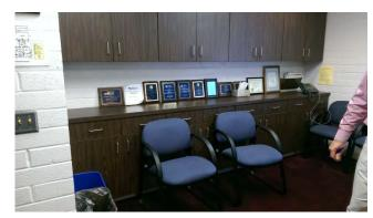
requires a 5-foot diameter turn around space. The existing cabinets are 36-inches tall; the height of the cabinets must not exceed 34 inches. The room is deficient in these areas.
