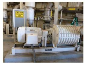
blowers have been rebuilt multiple times. Two other blowers are installed but have been taken out of service and are used for spare parts for the operating blowers. The condition assessment notes multiple improvements that c an b e m ade t o t he a eration p rocess a nd t he blowers t o i mprove p lant pe rformance and increase efficiency.
